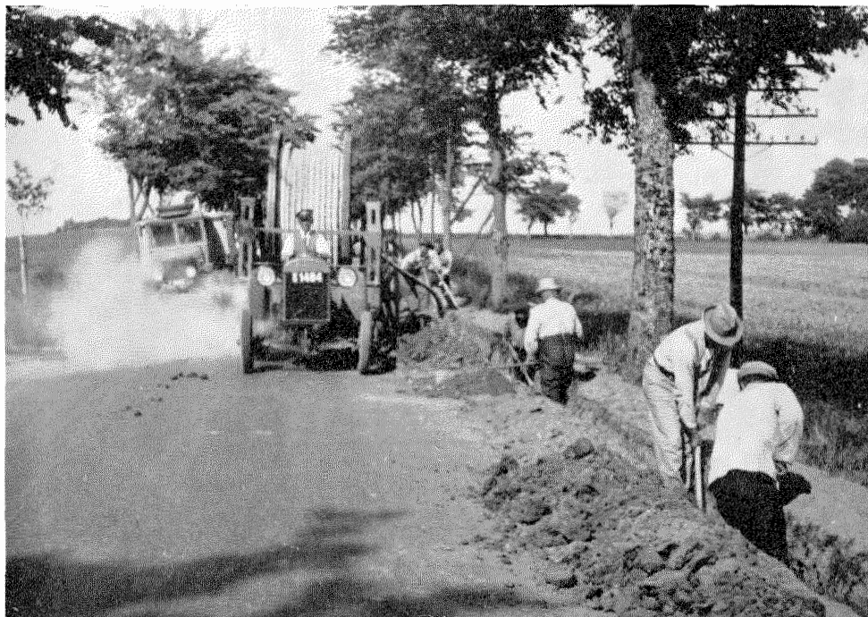
Figure 19—Transferring Cable to Trench Directly from Cart.
