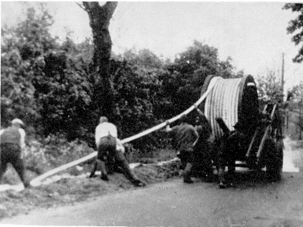
Figure 21—Unreeling the Cable Directly Into the Trench.
